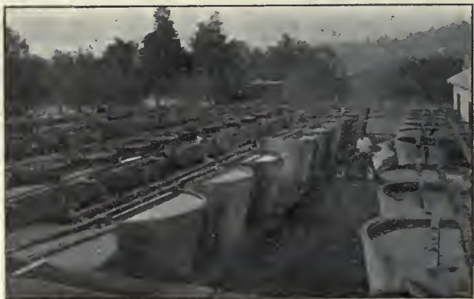
Unique Concrete Crystallizing Vats at Asti.
